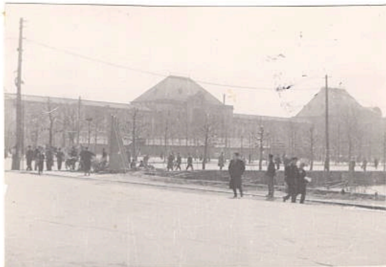
Tokyo Train Station
